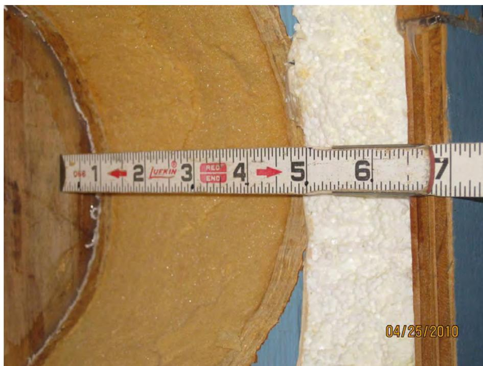
Figure 3. Big House wall material types and thicknesses.
